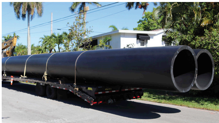
Above: A 54in diameter HDPE pipe - installed using HDD - won an award from PPE recently
