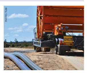
to irrigate 20,000 hectares of the Canterbury plains in New Zealand, for which the head contractor was Downer. For this, it has produced more than 170km of HDPE pipe using its mobile equipment.
