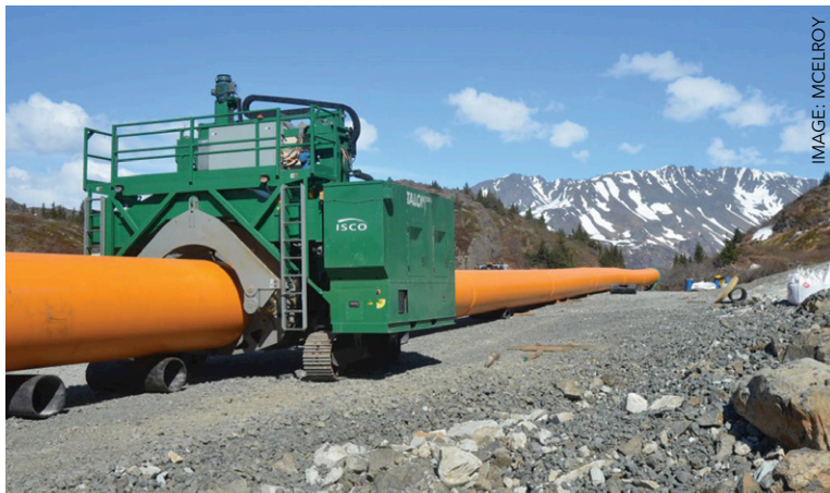
Above: McElroy's Talon fusion machine was used to join pipe sections for a hydropower project
