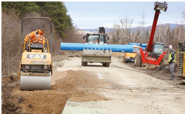
Above and right: Molecor's PVC-O pipe has been used to supply fresh water to Pernik in Bulgaria, after it suffered a severe drought
