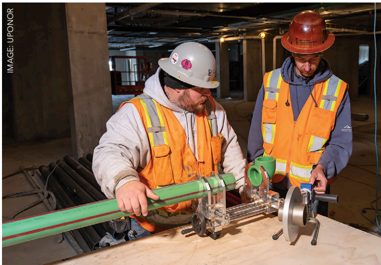
Above: Upponor says its PP-RCT pipe will help meet demand for commercial domestic water systems
