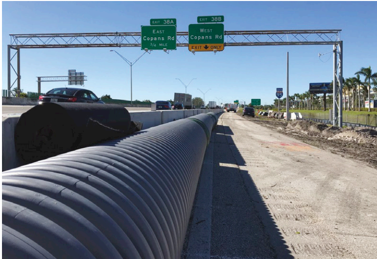
Above: Seven miles of ADS corrugated PP pipe has been installed on new express lane toll roads in Florida
