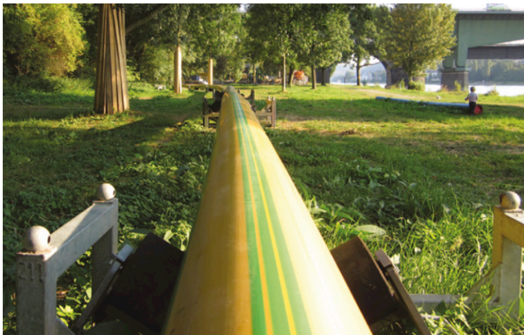
Above: Egeplast's SLA barrier pipe was recently installed into contaminated soil in Sweden using the HDD method
