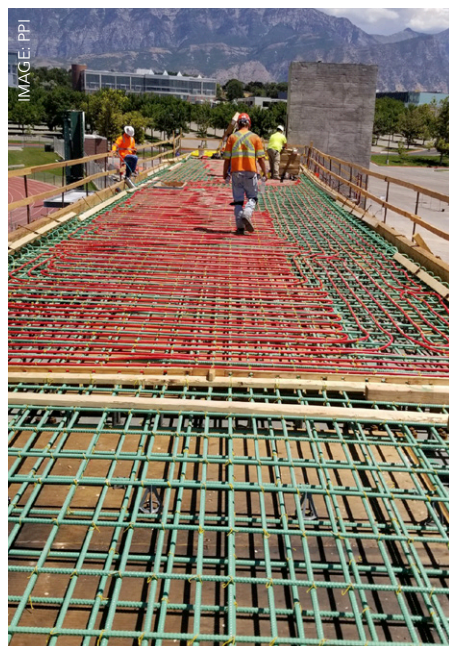
Loops of ‘snow melting’ PEX pipe were built into a pedestrian bridge in the USA
