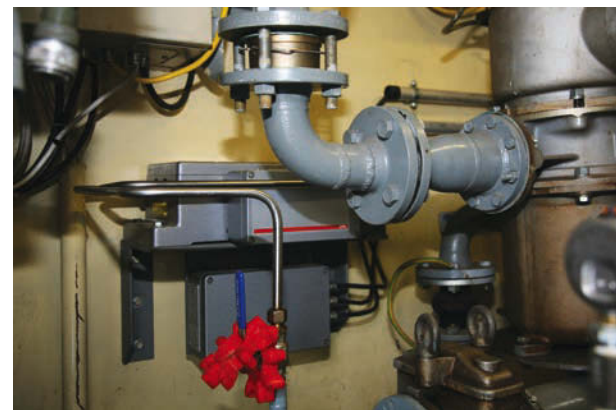
Figure 1. DPRn measuring cell with density sensor
