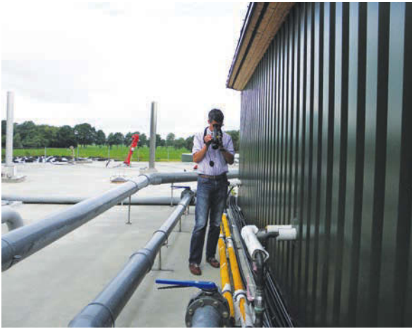
Explosion protected areas can be investigated from a safe distance with the FLIR GF320.
